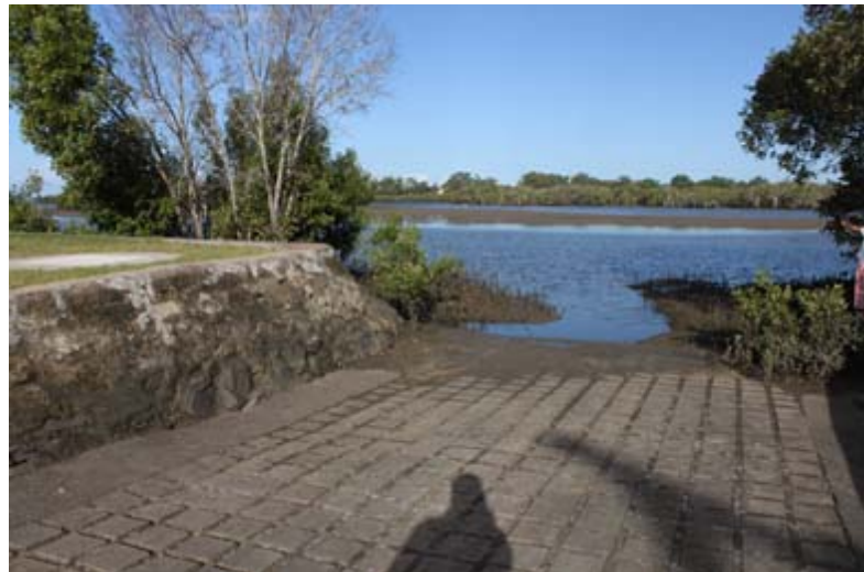
above: low water, The Esplanade ramp, Lota
