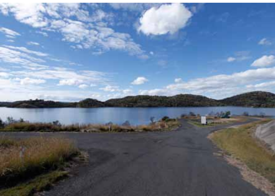
left: ramp view
