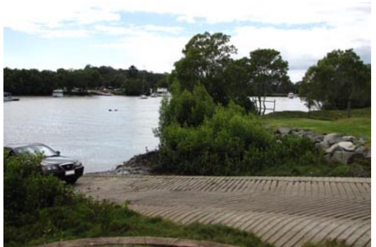
Alberton Road ramp, Riedel Road ramp across the river
