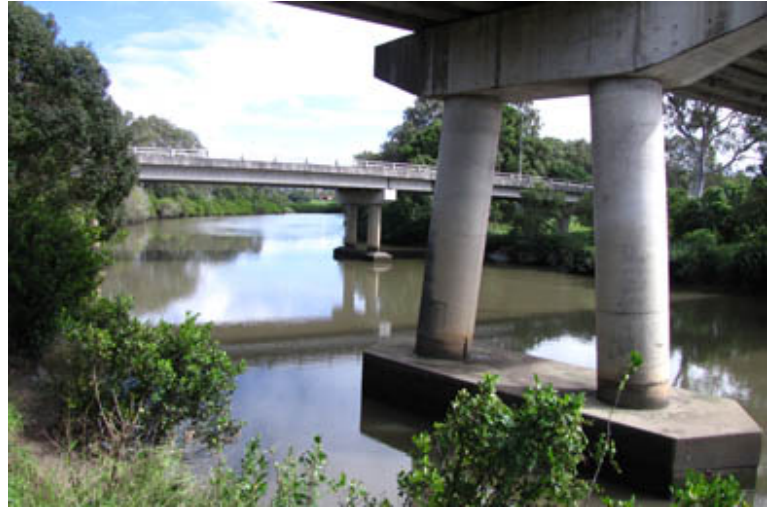
under the Pacific Highway bridges, Beenleigh
